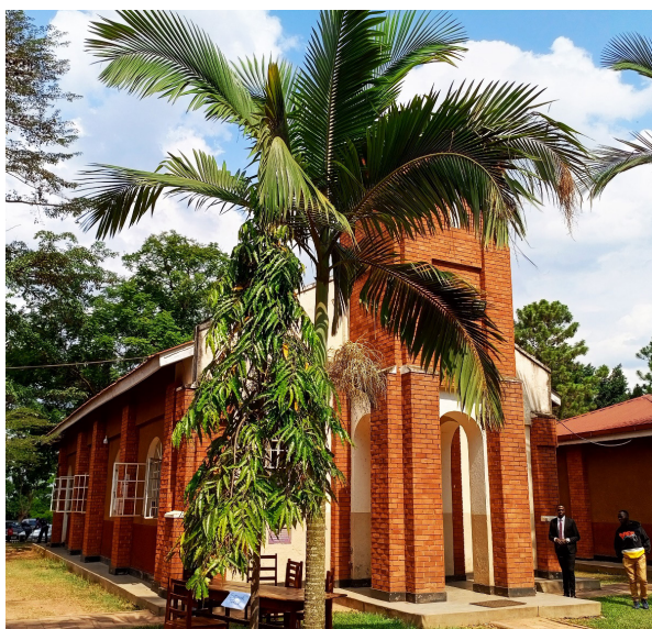
The exterior view of the current Chapel of St. Kizito Minor Seminary, Nandere, Kasana-Luweero Diocese.
